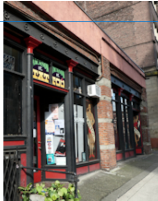
Figure xxx. Some buildings feature cast iron elements.
