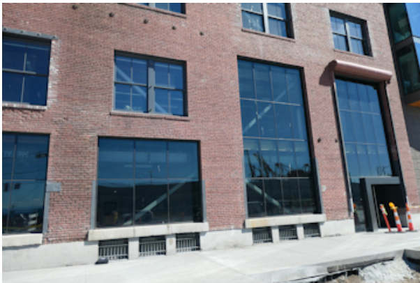
Figure xxx. The Alaskan Way facade of this building has been altered in an appropriate manner to accommodate new uses.
